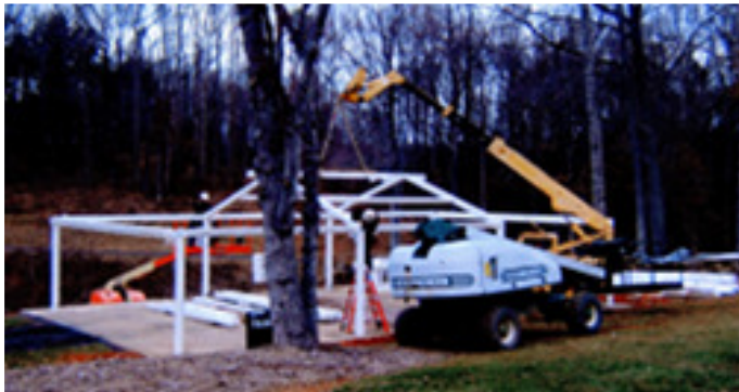
Picnic Shelter Being Built on top of Septic Repair Field
